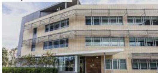
Building 8 – Dublin – Irlande
